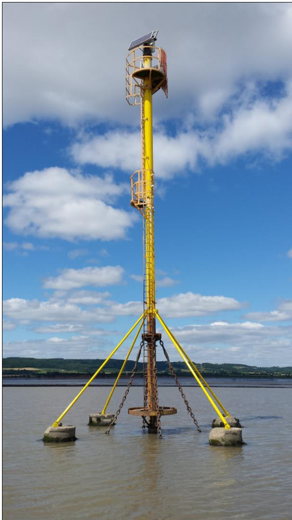
One of the beacons held in place by the new struts
