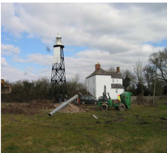
Work to dismantle old light in progress at Sheperdine
