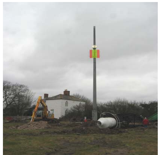
New lighting column in place
