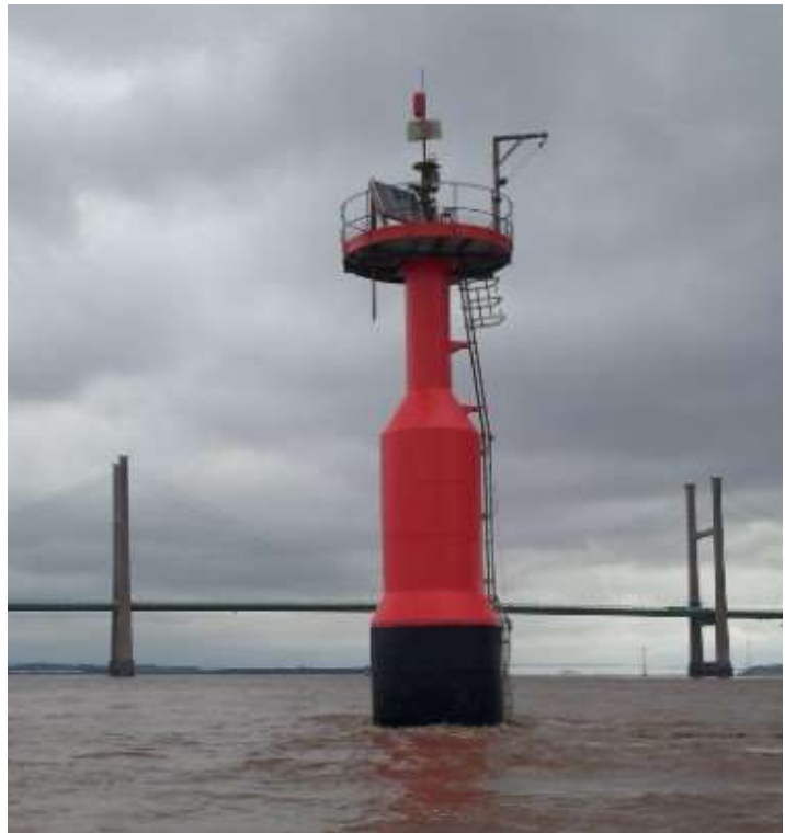
One of the beacons with its new coat of paint
