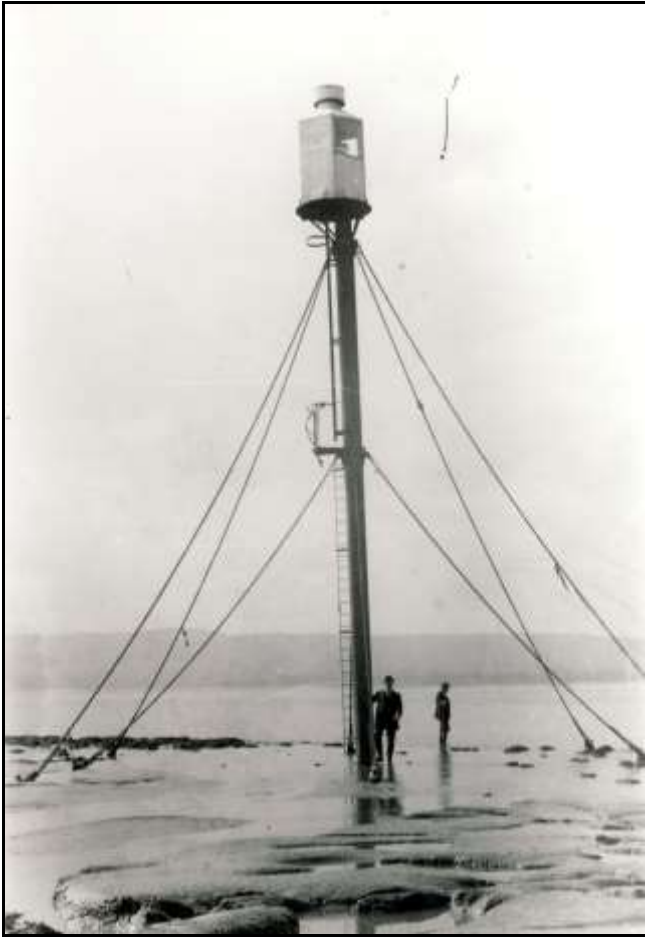
Oil lighting, early 1900s
