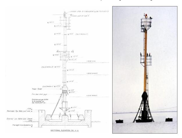
The gas lighting was replaced by solar panels and batteries in 1987 and following failure of the synchronising cable laid between the two beacons, l.e.d. lanterns featuring GPS synchronisation were fitted in December 2005.
