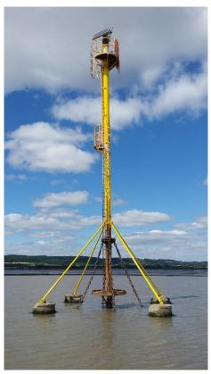
By the middle of 2017 welded joints at two of the legs at each beacon had failed as a result of the heavy vibrations set up by the vortices which developed around the legs in the fast flowing water. Temporary repairs were effected by installing sleeves over the affected joints, but a more permanent solution was required.
