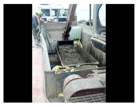
The concrete was mixed in a skip (left) aboard the 'Riparian' in batches of about 5 tonnes.
