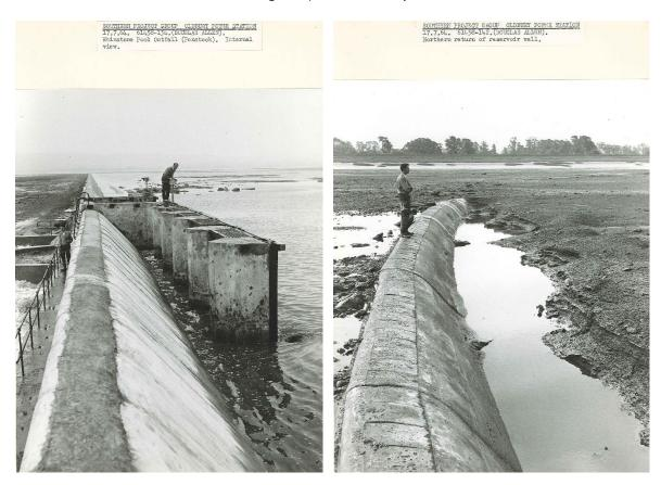
The wall would retain a depth of water of up to 1.2m which would keep the power station supplied with cooling water during periods of low tide.
