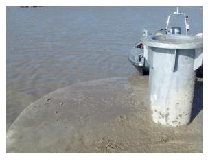
The base formwork, fabricated by Sharpness Shipyard, included a means of adjusting and maintaining the flanged stub in a vertical position during the concrete pour. The bases were positioned carefully to ensure that the new beacons would be exactly aligned on the required navigational bearing.
