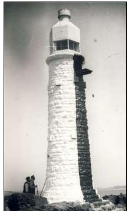
The photograph (*right*) taken in the early 1900s shows the original shape of the lantern housing and tapered base of the stone tower erected by the railway company. The base has since been concreted over.
