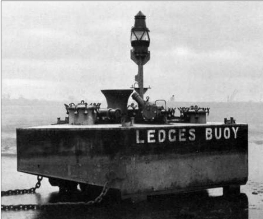
Ledges Buoy as installed in 1961 showing pockets for the dissolved acetylene gas and CO<sub>2</sub> cylinders, bell and lantern.
