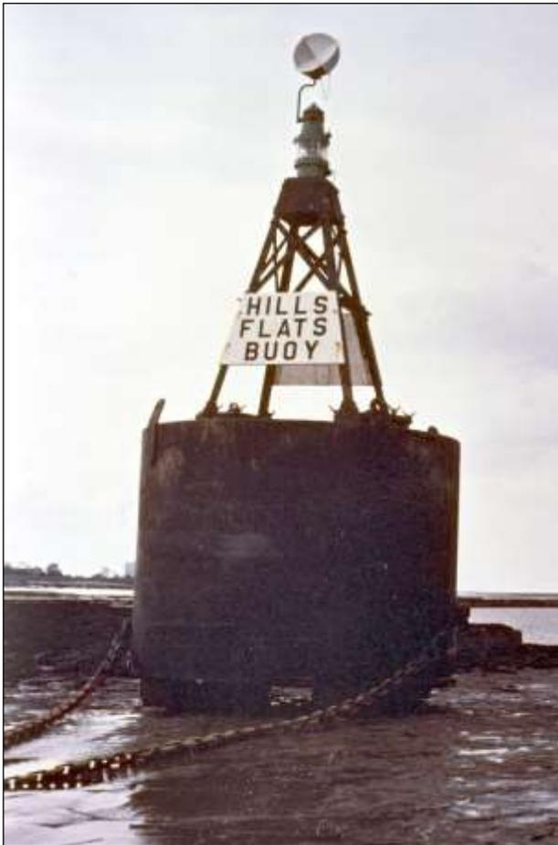
An unlit iron buoy was substituted in April 1905. The present green can buoy, installed in 1961, was fitted with gas lighting (pictured left). Conversion to solar power and battery was made in 1987.
