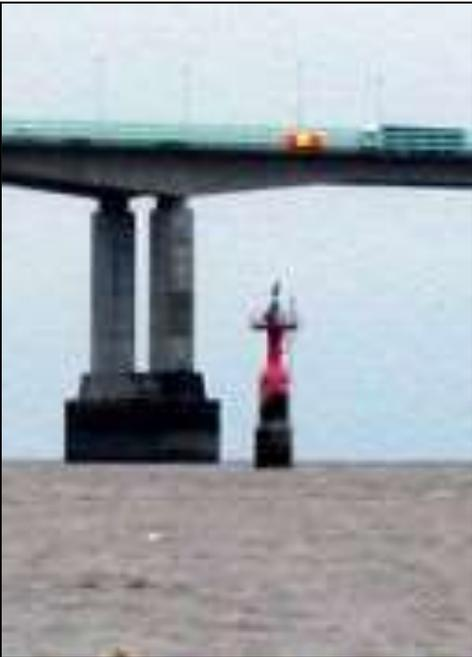
A mark and light which, when aligned with the Lady Bench beacon, define part of the track between the Severn Bridge and the Second Severn Crossing are provided on the Second Severn Crossing.
