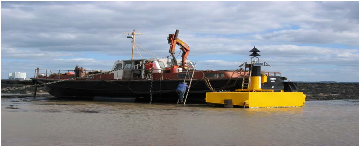
Buoy maintenance works, River Severn
