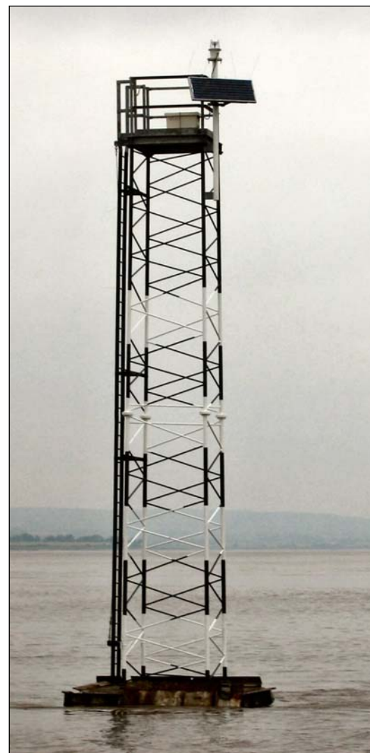
New tower completed
