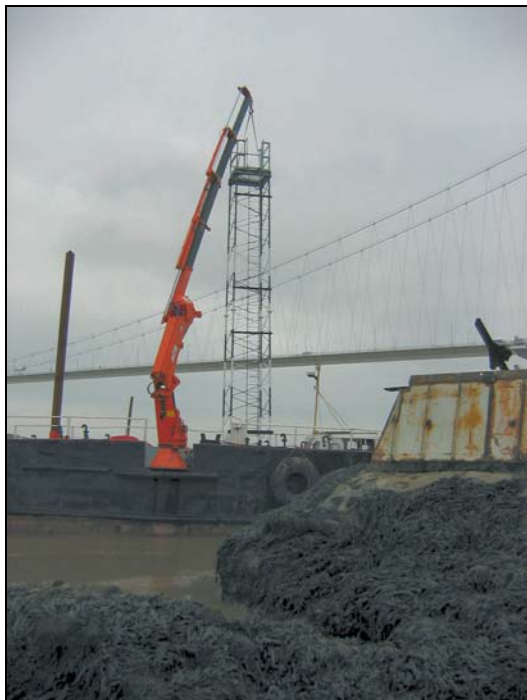
New tower being craned into position
