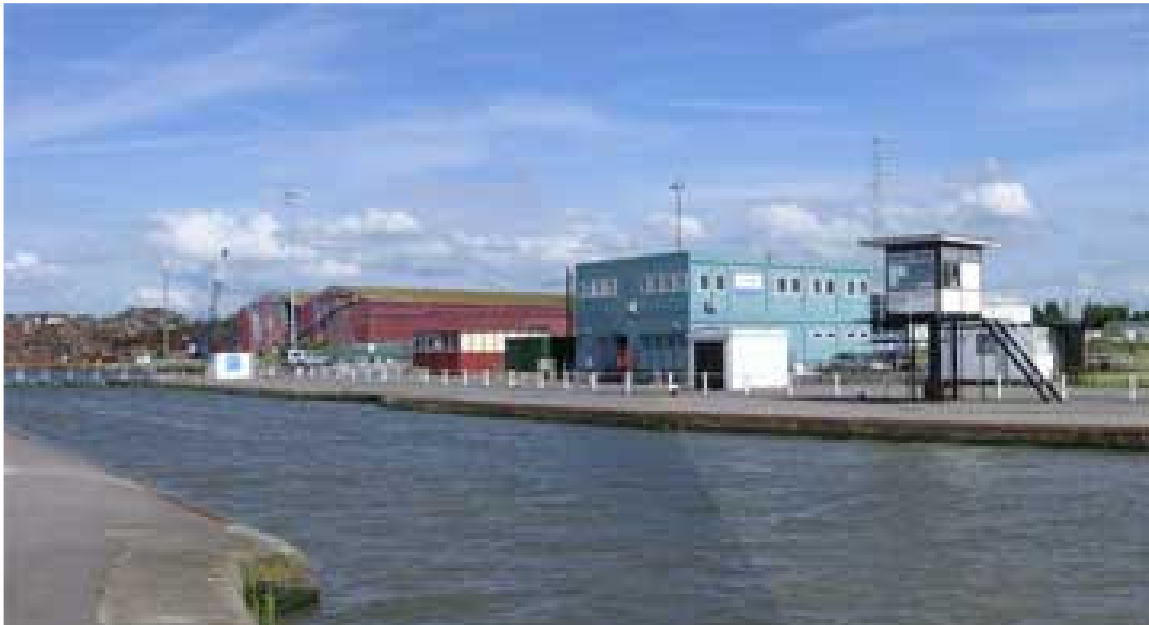
GHT's office at Sharpness Dock (part of blue building)
