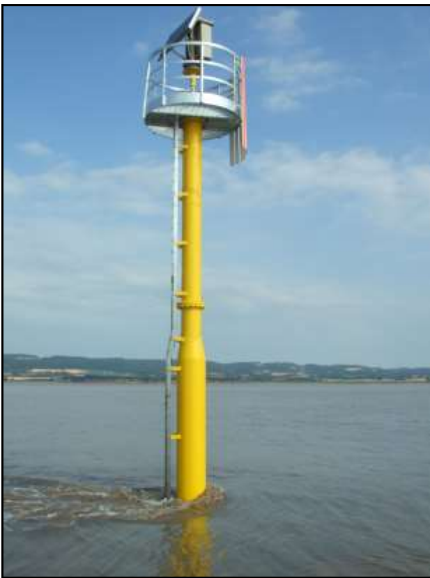
Front mast (July 2018)
