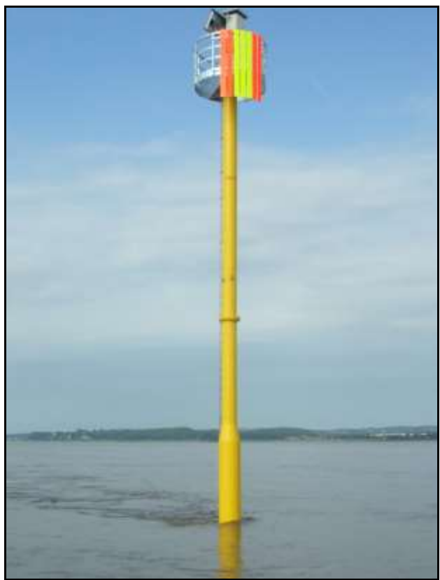
Rear mast (July 2018)
