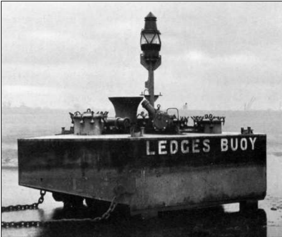
Ledges Buoy as installed in 1961 showing pockets for the dissolved acetylene gas and CO 2 cylinders, bell and lantern.
