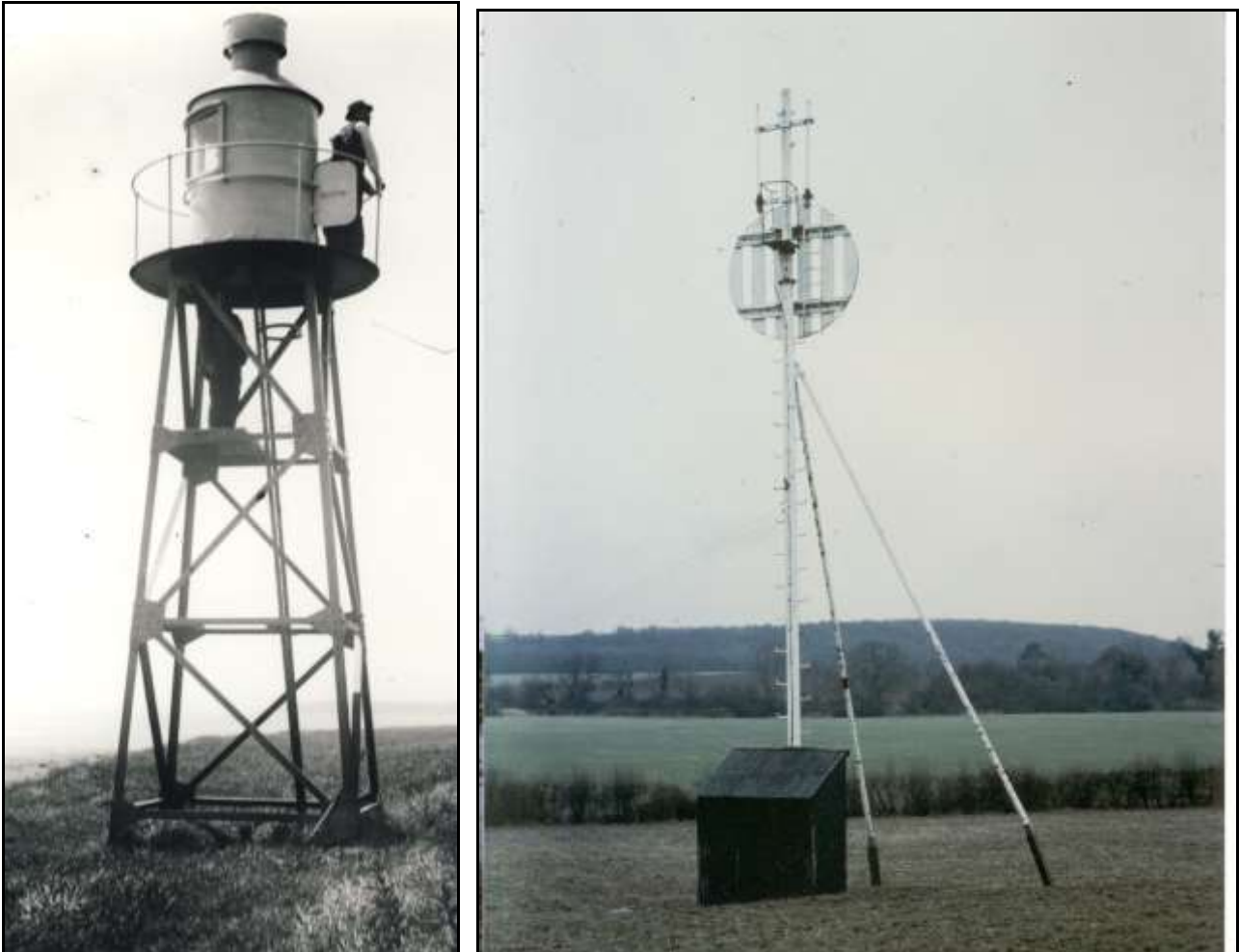
Inward Rocks: Front light (post-1907) and rear beacon (viewed from the NE) following electrification in 1962.
