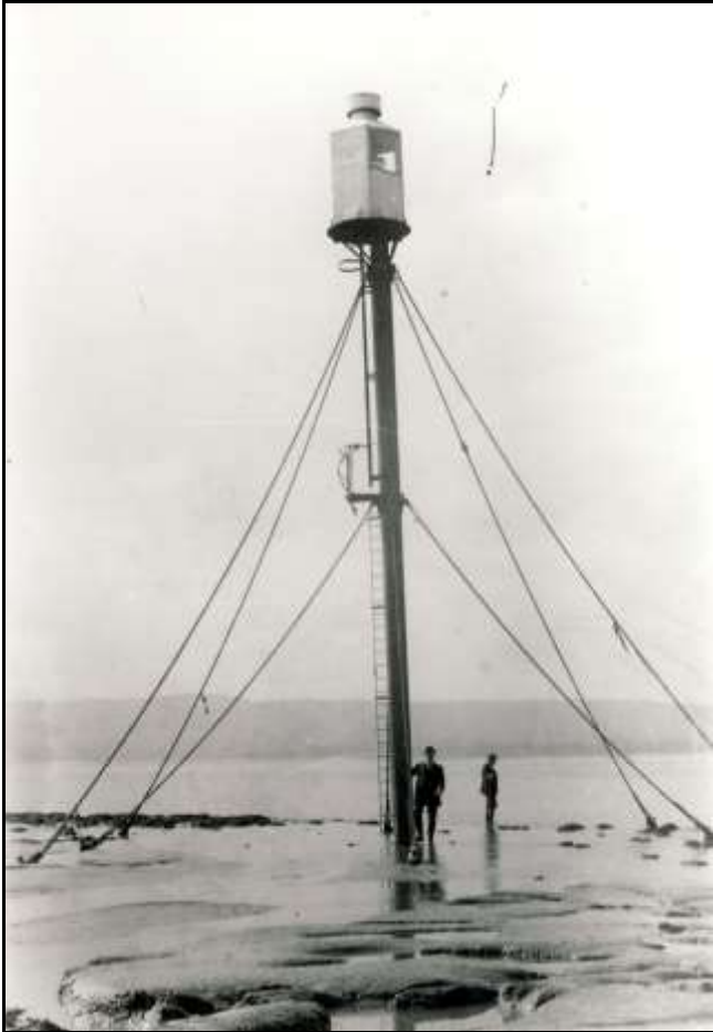
Oil lighting, early 1900s
