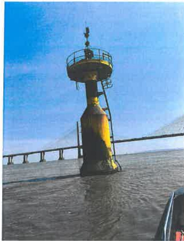
Lower Shoots Beacon – inspection pre-maintenance March 2021
